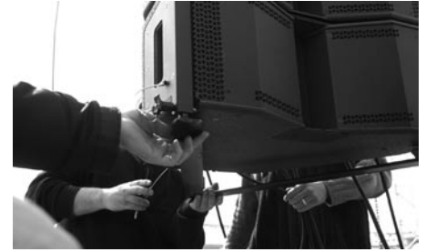
Figure 18: Mounting the bottom rigging frame
