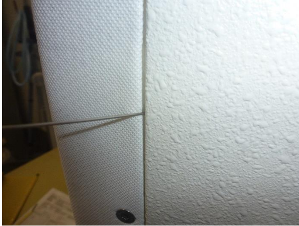
1. Penetration with the access probe \varnothing 1mm not possible
